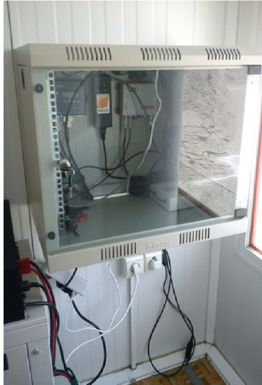
Figure 4: some of the communication network equipments of TPSL site inside a rack
