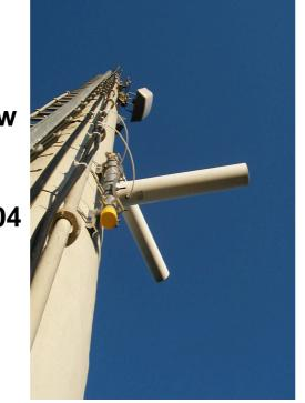
Fig 3: WLAN repeater
